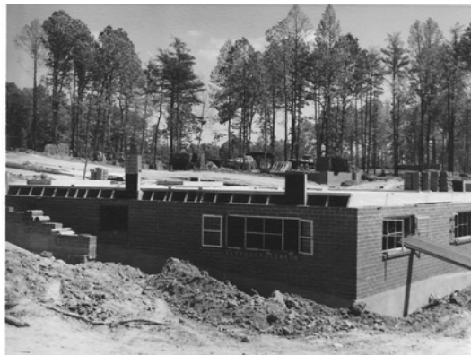
Photo: RF exterior basement May 11, 1963
