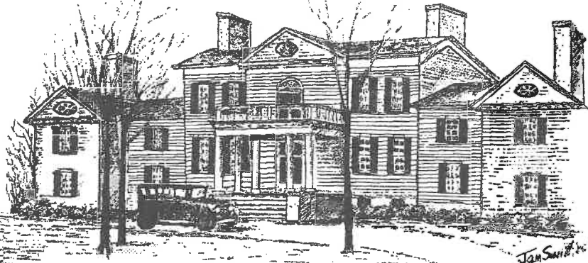
MANOR HOUSE 1796-1925 RAVENSWORTH PLANTATION, VA.
